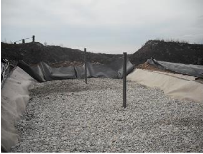
Figure 5. Gravel drainage layer.
