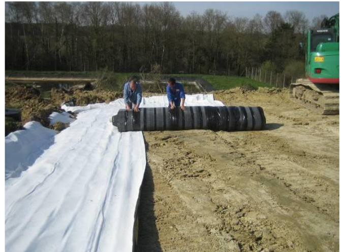
Figure 15. Drainage Geocomposite Installation.
