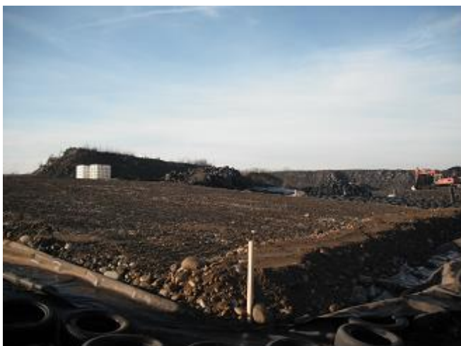
Figure 3. Pad graded with a 5% slope.
