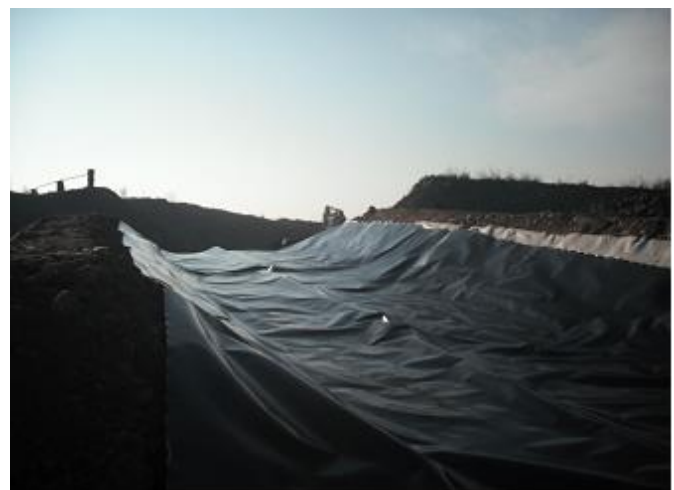
Figure 4. Geomembrane Installation.
